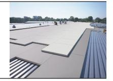
When a multiple layer insulation application is used, the joints of the insulation boards in the top layer should be vertically staggered and offset a minimum of 6.0" from the joints in the insulation boards in the layer below.
