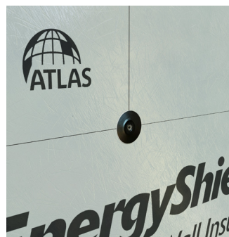
Figure 2: A single washer-style fastener can be used to bridge adjacent insulation boards.
